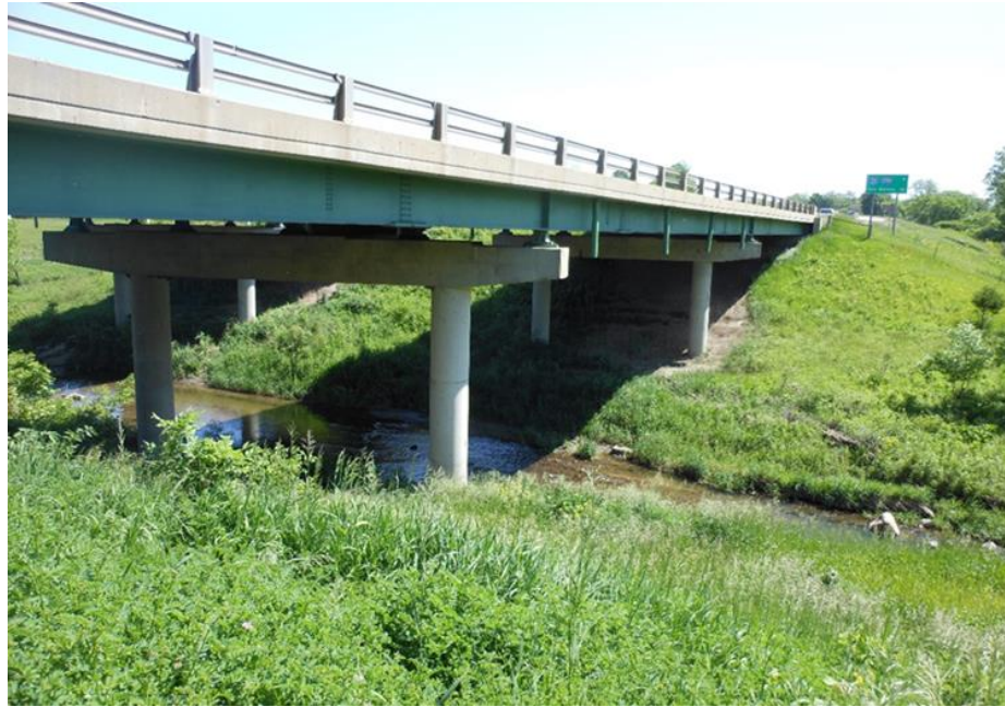
Figure 3.1. I-80 Bridge, on Interstate 80 over Sugar Creek
